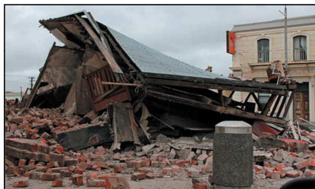
Figure 5. Total destruction of a brick building along the main road into town.
