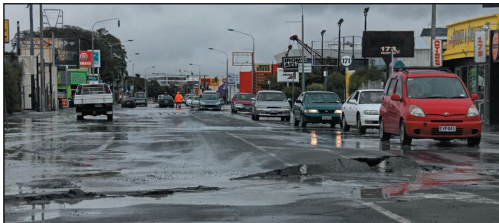
Figure 4. A road cracked and heaved, and then flooded by a burst water main.
